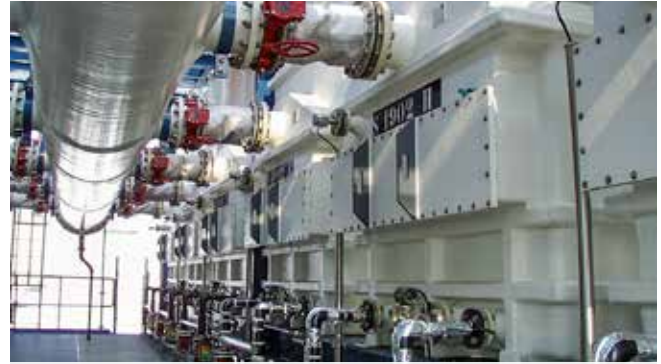
HOK adsorber, detailed view
