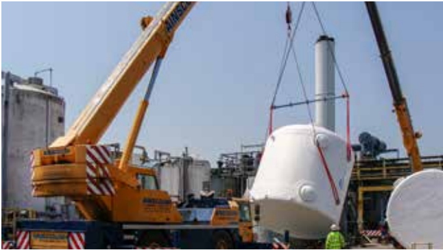
HOK adsorber, installation
