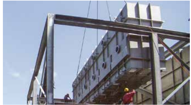
HOK adsorber, installation
